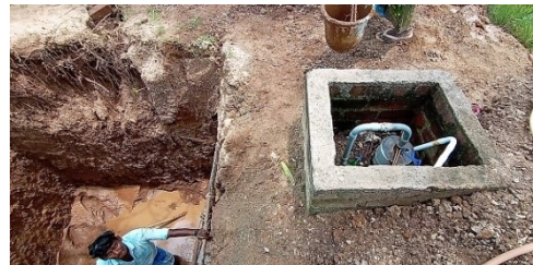
Photo 3: Capped Well Head
