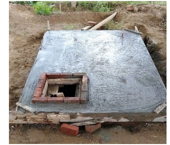
Photo 5: Tank with roof
