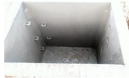
Photo 4: Concrete leak-proof tank
